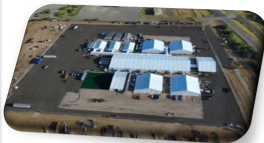
Figure 7: Soft-Sided Facility at Laredo, Texas
