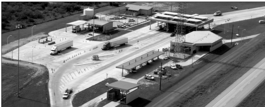
Permanent checkpoint, Laredo sector
