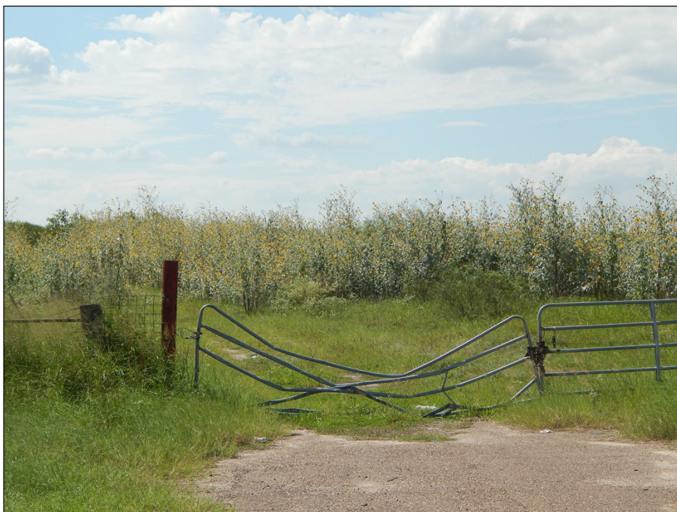
Figure 13: Mangled Gate Suspected to Have Been Caused by Illegal Border Crossers along Highway 281 in Brooks County, Texas
